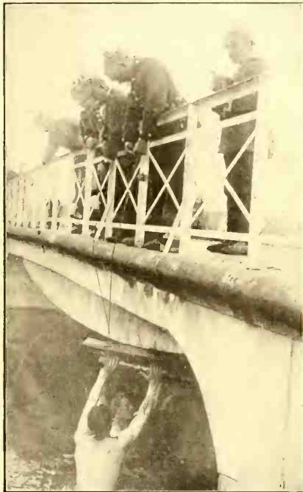
Photos Copyright by Underwood & Underwood. German Military Engineers Engaged in Mining a Bridge. At the Push of an Electric Button This Mighty Structure Will Be Blown to Atoms.
